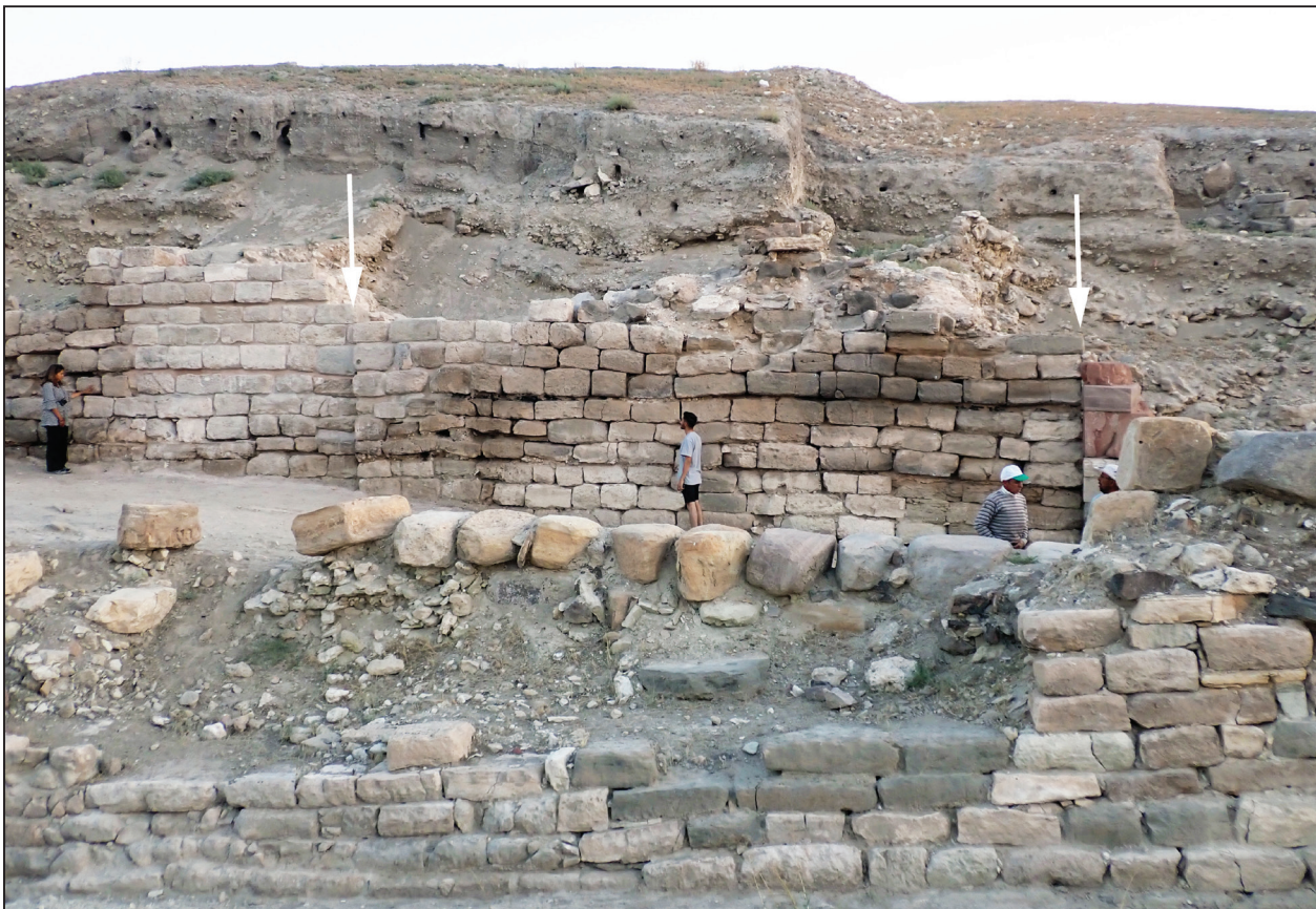
Fig. 9. The newly conserved north wall of the South Gate (9th century B.C.). The arrows indicate vertical offsets in the wall. A glacis, or stepped terrace wall, is in the foreground. (Photo by Brian Rose; courtesy Penn Museum, Gordion Project Archives.)
