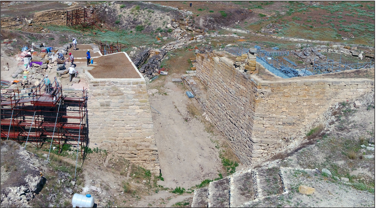
Fig. 5. The restored East Citadel Gate (9th century B.C.), at the end of the 2019 season, looking northwest. (Photo by Braden Cordivari; courtesy Penn Museum, Gordion Project Archives.)
