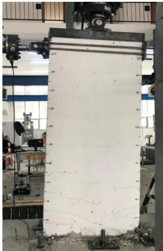
Figure 7. Post-Experiment View of the Reference Reinforced Concrete Shear.
