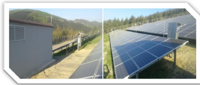
Figure 1. Image of the partially shaded PV array.
