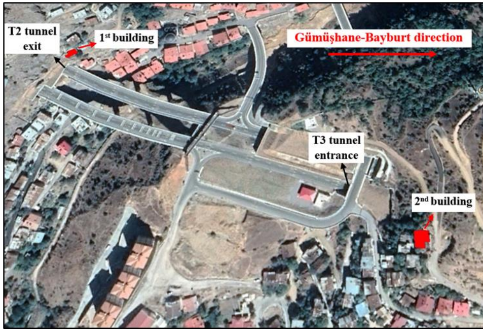
Figure 4. Satellite image of the buildings
