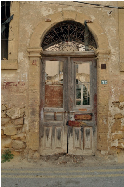
Photograph 2. An old door of a ruined house, Nicosia Walled City.
