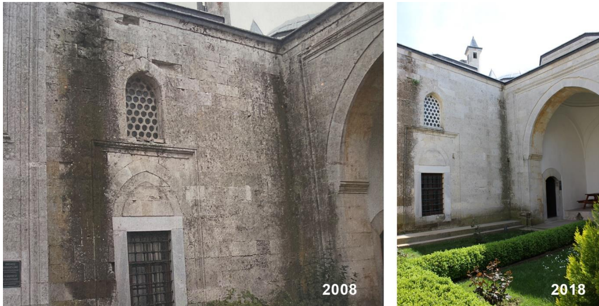
Figure 6 - Before (2008) and after (2018) facade cleaning.
