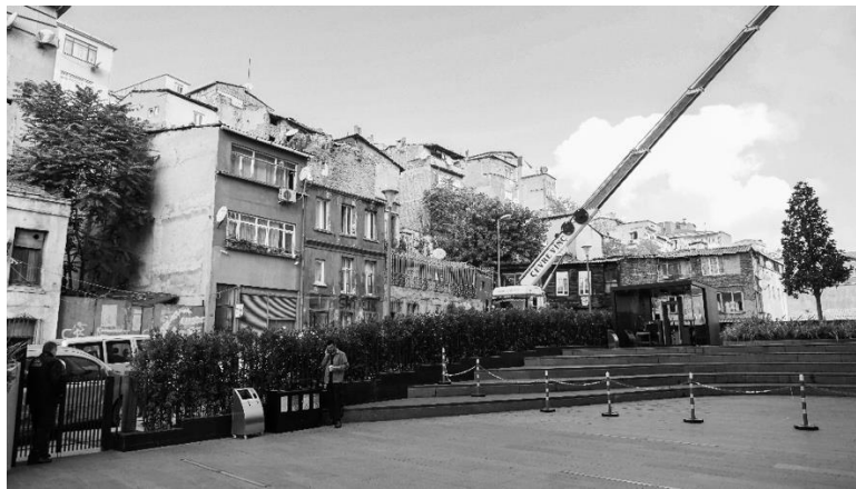
Figure 8 - The limits between the surrounding urban context and the rear part of the podium of Arter (Photographed by the authors).
