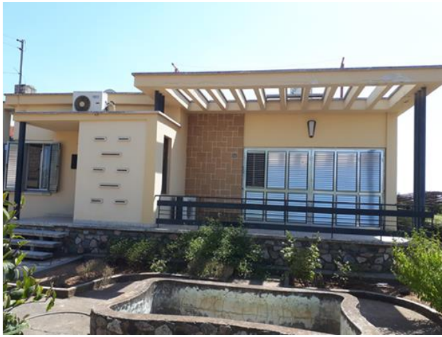
Figure 21 - Open and semi-open space examples of modern houses in Güzelyurt (Source: Authors).
