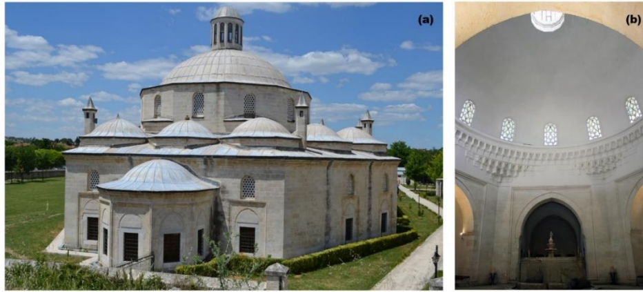
Figure 4 - Building masonry wall (a), plastered interior walls and dome (b).
