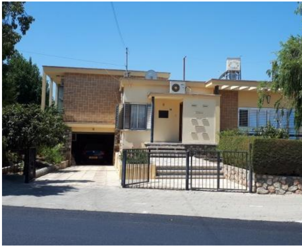
Figure 8 – A Front façade of a modern house in Güzelyurt (Authors, 2021).
