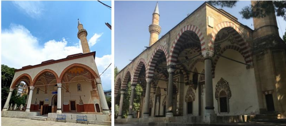
Figure 2 - Exterior views of Yeni Mosque (left) and Sultan Mosque (right).
