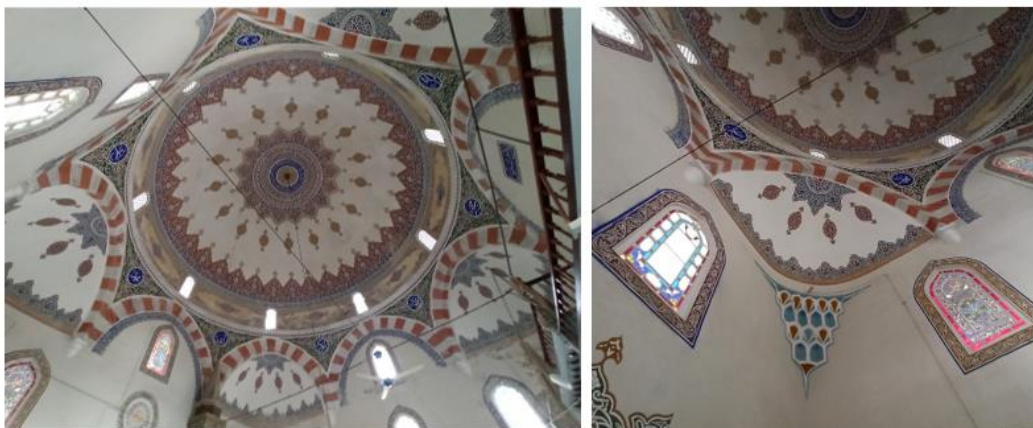
Figure 3 - Main dome and transition elements in the Yeni Mosque.
