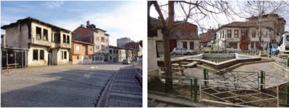
F. 2: The general views of main street and historic town center of Orhaneli (Güneş Kaya, 2017)
