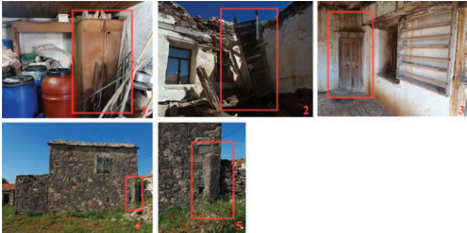
F. 9: 1: Yunak with cupboard in H2. 2: Yunak as wooden cabinet in H12. 3: Yunak as a niche in H14. 4: Water outlet of yunak in H14. 5: Close view to water outlet of the yunak in H14.
