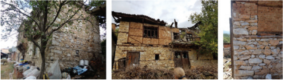
F. 10: Stone masonry walls that continue on the upper floor in Serçeler village (Güneş Kaya, 2018 and 2020) and detail of a continuous stone masonry wall (Güneş Kaya, 2018)
