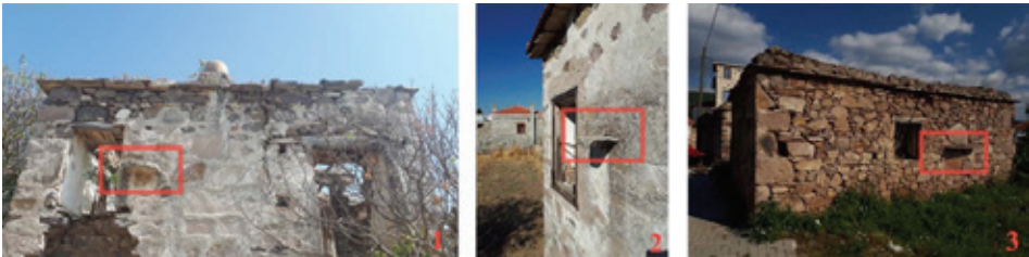
F. 15: 1: Exterior shelf in H3. 2: Exterior shelf in H5. 3: Exterior shelf in H13. (Photos by Sarıbekiroğlu, 2017)
