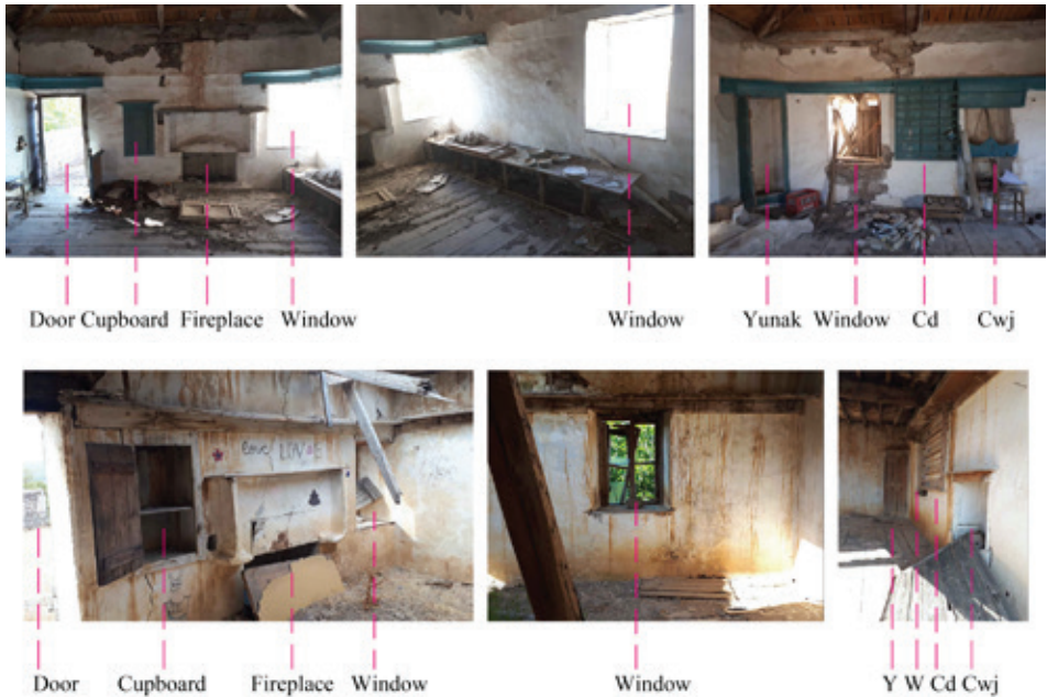
F. 4: Living spaces of H5 and H14 at first level. Above photos belong to H5 and below ones to H14. Left: West walls. Middle: North walls. Right: South walls. Y: yunak. W: window. Cd: cupboard for dishware. Cwj: cupboard for water jugs (Photos by Saribekiroğlu, 2017; prepared by Saribekiroğlu, 2022)
