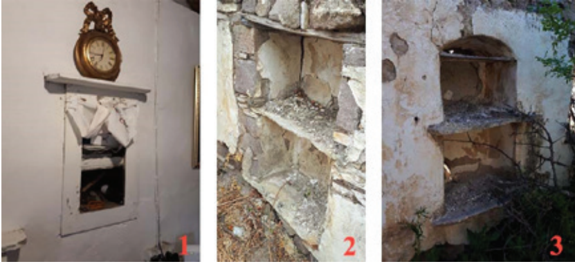
F. 11: 1: Niche with shelf on top in H7. 2: Niche in H11. 3: Niche with arched top in H13. (Photos by Sarıbekiroğlu, 2017, 2020)
