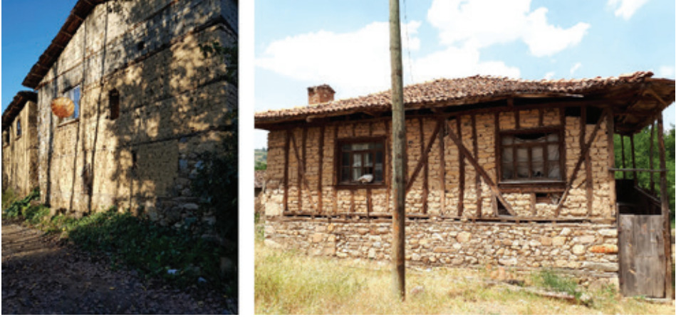
F. 9: An adobe masonry ground floor in Kusumlar village (Güneş Kaya, 2019) and a stone masonry ground floor in Sadağı village (Güneş Kaya, 2018)
