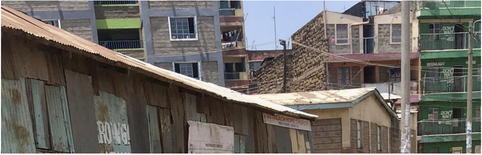
Figure 5: The Various Structures in the Valley Today
