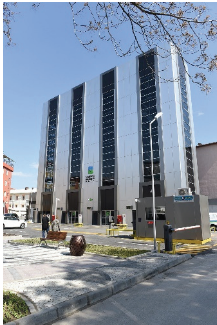
Fig. 1 - Automated multi-story parking garage with 4 units (Balıkesir, Turkey)
