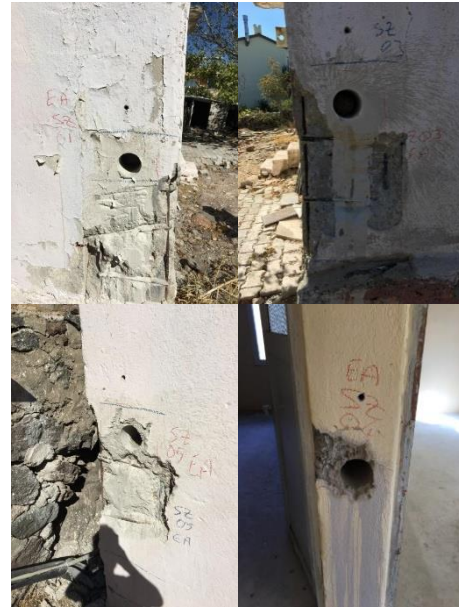
Figure 4. Column stripping and core concrete, existing building
