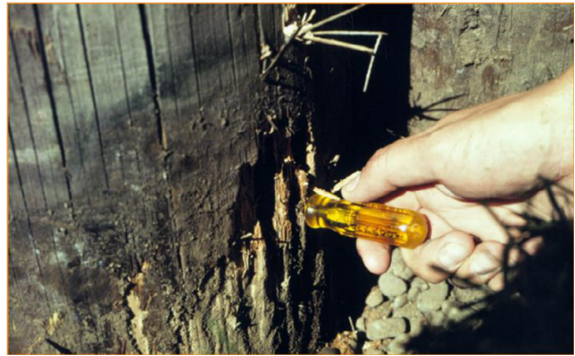
Figure 1. Example of soft rot damage on the surface of an untreated Douglas-fir pole.
