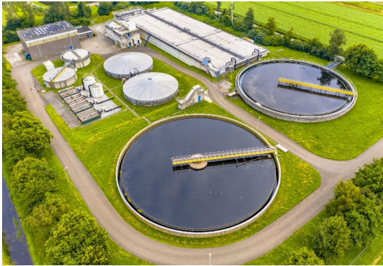
Figure 3. View of a sample wastewater treatment plant
