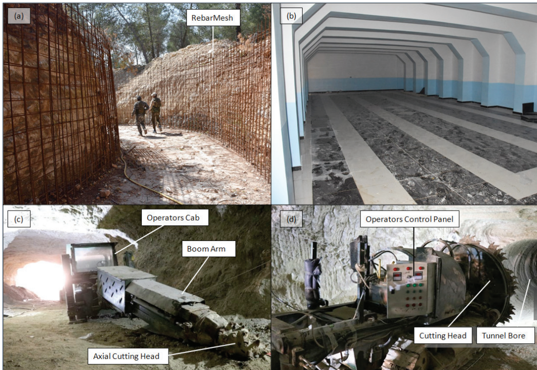
Figure 6. (a). Entrance to an SDF, YPG and YPJ underground facility in the mountains around Afrin showing vertical and horizontal rebar wired in a grid pattern ready for concrete to be poured or sprayed 127 . (b). Reinforced room in an SDF, YPG and YPJ underground facility located in the mountains around Afrin containing multiple one hundred meter long tunnels 128 . (c). Front left view of an extendable and multi-axial boom-mounted cutting head machine captured in-situ in a subterranean structure in the mountains around Afrin 129 . (d). Rear right side view of an ITTBM captured in-situ in a subterranean structure in the mountains around Afrin 130 .
