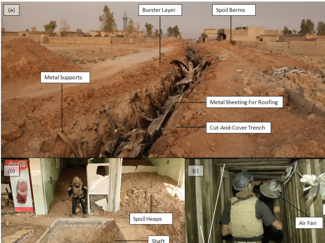
Figure 3. (a). Covered trench outside Bazwaia, in Ninevah Province with the metal supports and roofing visible that was used as the roofing 118 . (b). Shaft entrance to a tunnel inside a building in Bazwaia 119 . (c). Tunnel below the shaft identified in image (b) showing shoring on the wall and roof as well as power and ventilation 120 .
