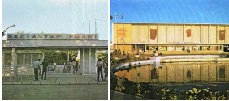
Figure 31. Gaziantep Fairground, Fair Building, 1982 (URL-15)
