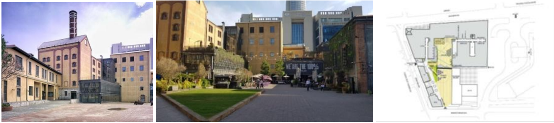
Figure 5. Bomonti Beer Factory Before and After Restoration (URL-2)
