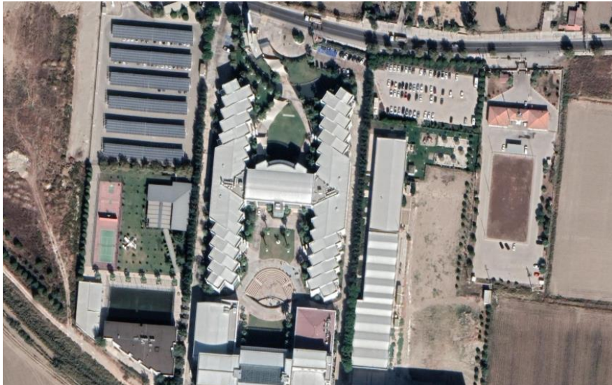
Figure 2. Satellite image of İzmir Bakırçay University main Campus.
