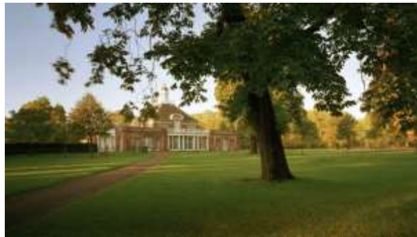
Şekil 6. Kensington Gardens da bulunan serpentine gallery yapısı görseli, Kensington Gardens, Londra (Figure 6. Image of serpentine gallery structure in Kensington Gardens, Kensington Gardens, London)
