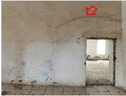
Figure 9. The stone wall, which was built later, that provides the transition to 1-03 office room on the northeast facade wall of 1-01 Entrance-Hall
