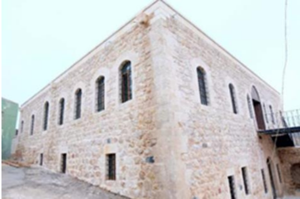
Figure 2. Images of Derik former government building
