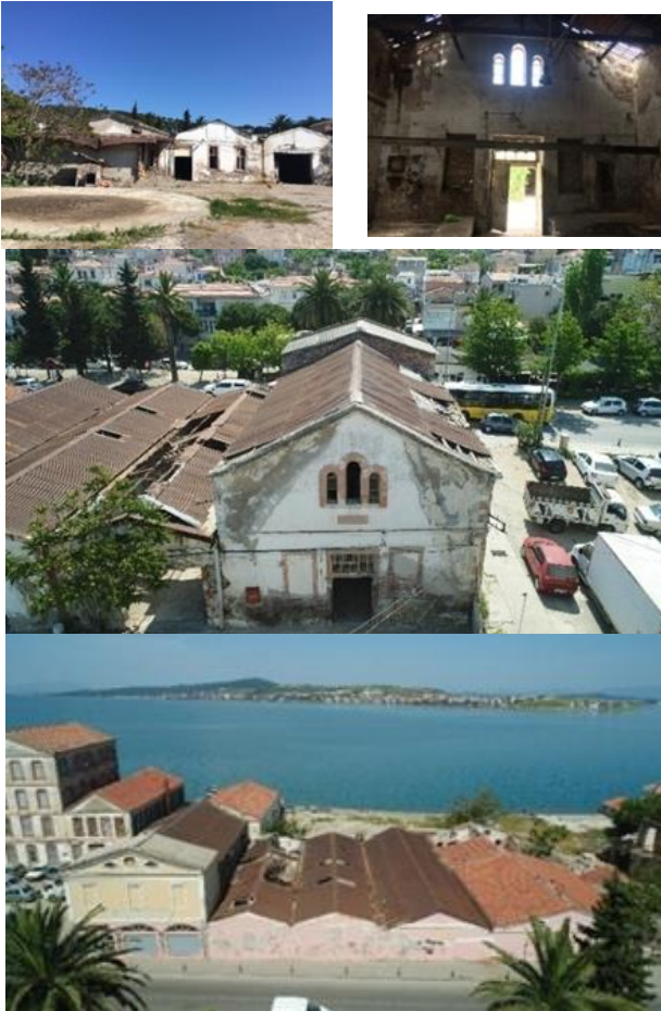
Figure 3. Tariş olive oil factory building stock indoor and outdoor
