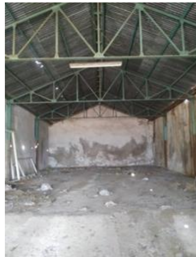
Figure 9. Iron profiles and beams along the long side of the structure
