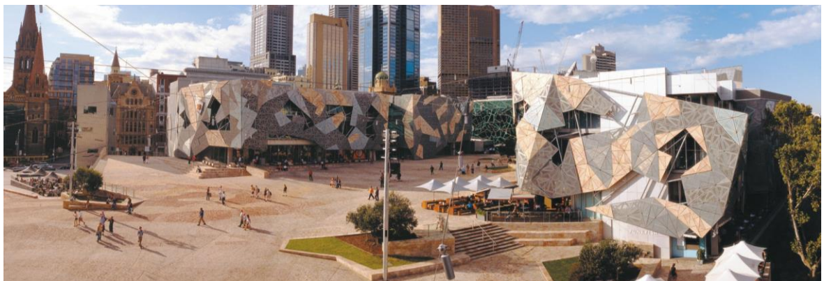
Figure 9. Fractal geometry in the Federation Square façade panel design (Osama et al., 2014)
