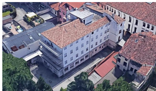
Figure 6. Ospedale Civile Building, old view (Google Earth, 2022)
