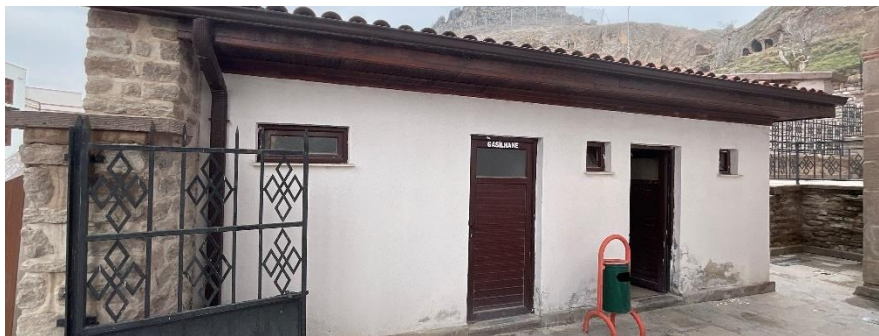
Figure 17. The view of the structure consisting of a funeral washing room, ablution area, toilet, and washbasin
