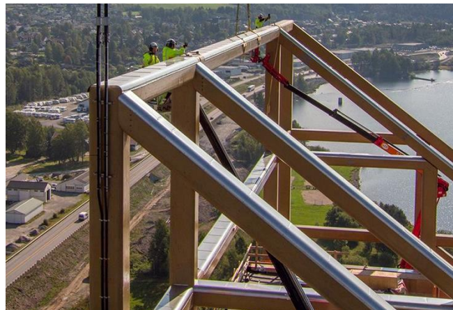
Figure 2. Metal caps for the top frame (CTBUH, 2021) (Photo: Moelven)
