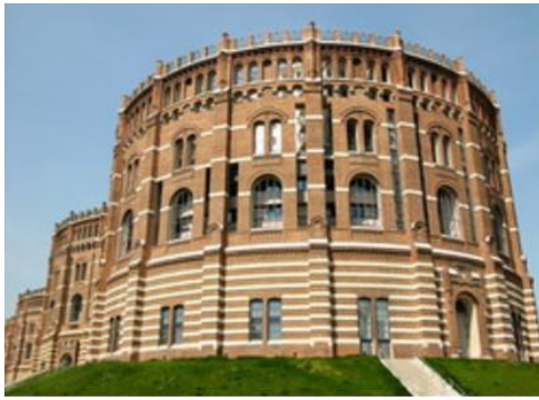
Figure 16. A view of Gazometre D from the south, showing the arrangement of openings and their relationships within the Gazometer structures (www.gasometer.org, June 2005).
