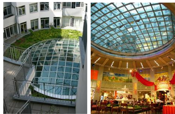
Figure 13. The overall views of the transparent superstructure created in the inner courtyard of Gazometre C structure from the inside and outside (www.gasometer.org, June 2005).
