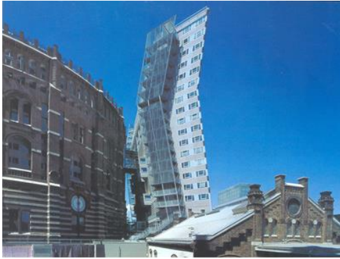
Figure 11. The relationship between Gazometre B structure and the shield-like new extension (Himmelb(I)au C., 2003).
