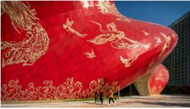
Figure 7. Facade , is made of perforated aluminum to support its flexibility and curved form, and it is painted in red, representing Chinese culture and art. Reference: Steven Chilton Architects.
