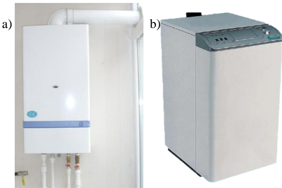
Figure 3. Individual heating system devices a) Combi boiler [22], b) Floor heating [23]
