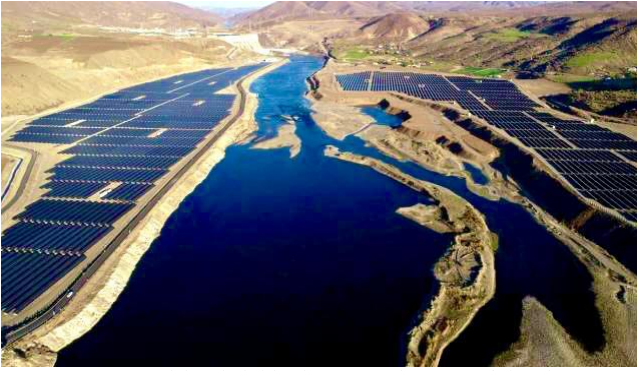
Figure 2. Aşağı Kaleköy hybrid solar power plant (Genç/Bingöl-500MW) [13].
