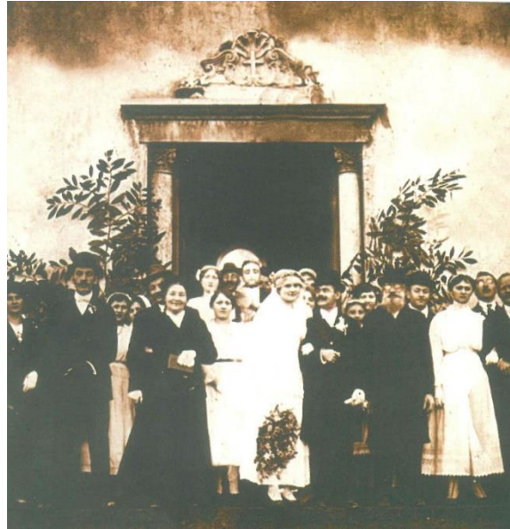
Figure 19 - North façade of the church-1918 (Adamska, 2004, p.28)
