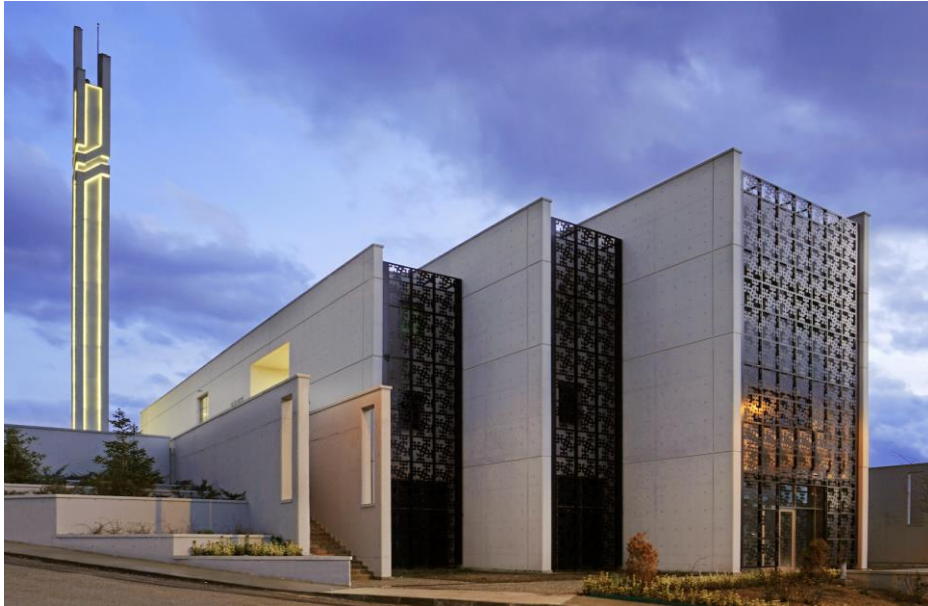
Fig. 12 - Looking at Salih Bezci Mosque Complex from a west-northwest direction.
