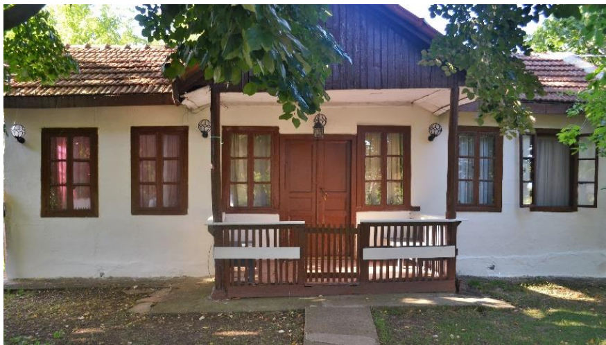
Figure 5 - The current situation of the house in Figure 4 (Salihoğlu, 2019).
