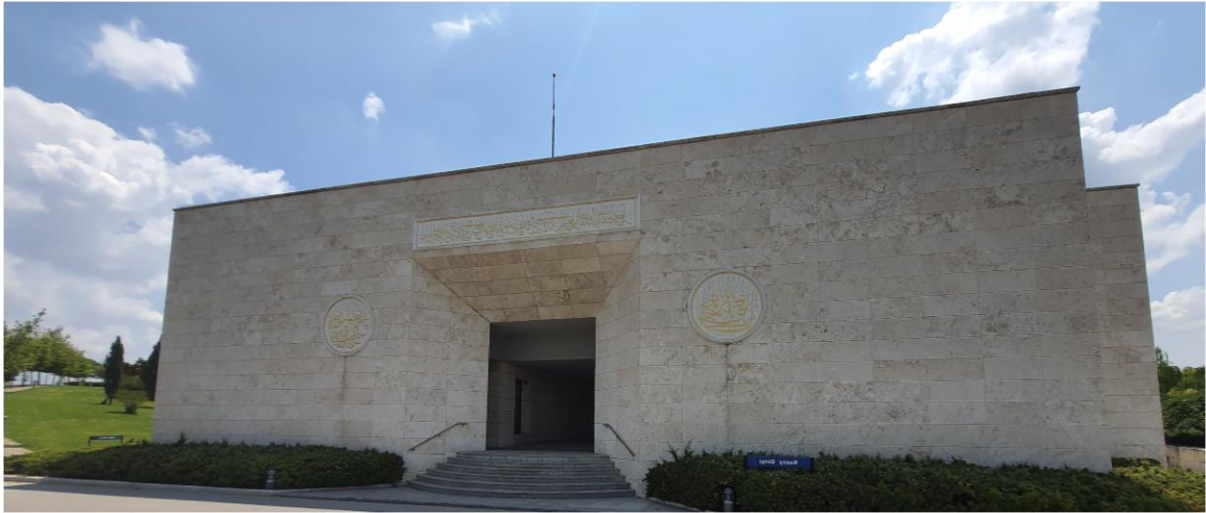
Fig. 8 - A view of the monumental entrance of Doğramacızade Ali Pasha Mosque. The user loses the connection with the rest of the building.
