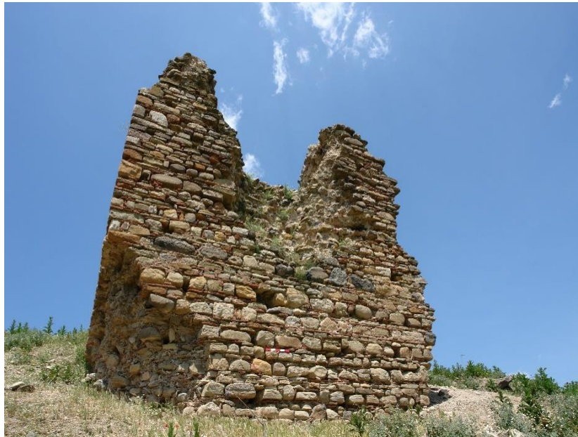
Figure 5: The concealed Course Technique on the Fortress Wall
