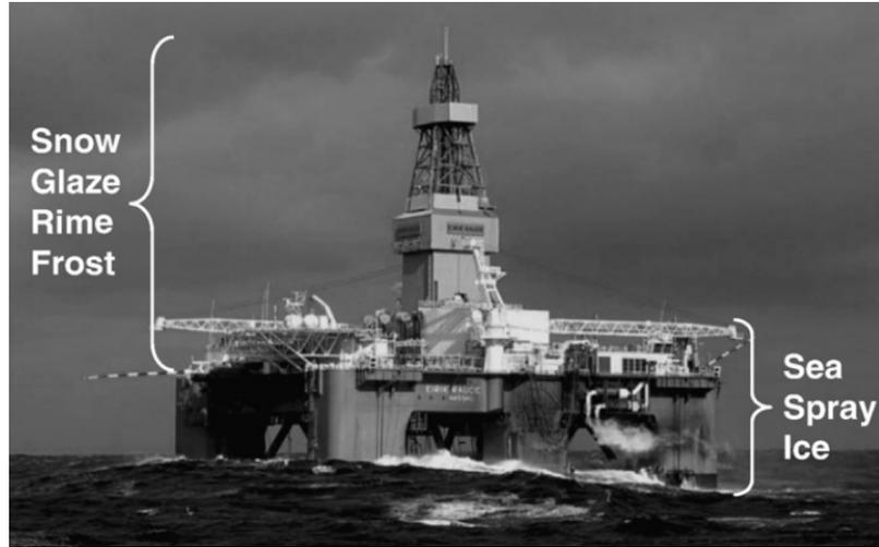
**Figure 3.** Icing effects on offshore structures [15].
