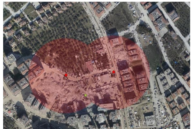
Figure 6. The debris of the "rönesans residence "
