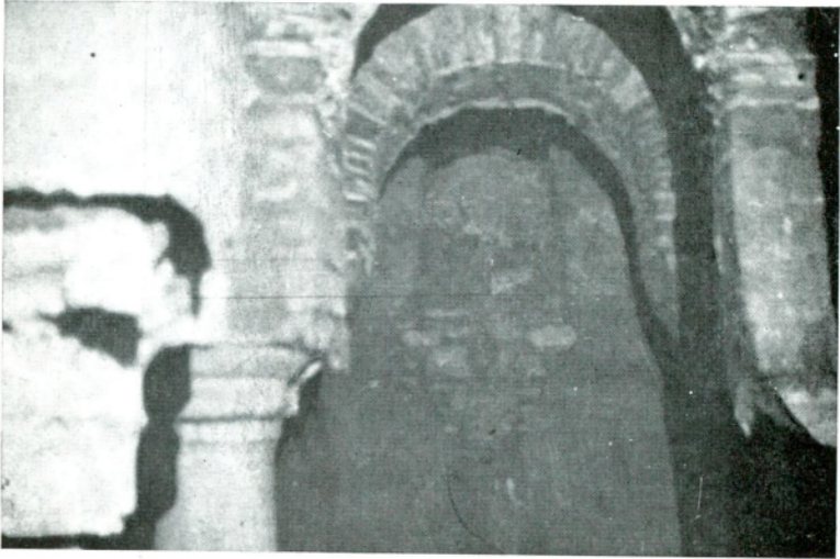
Res. 28 — Sarnıca vaktiyle ışık veren pencere yeri. Fig. 28 — Window opening which formerly gave light to the cistern.
