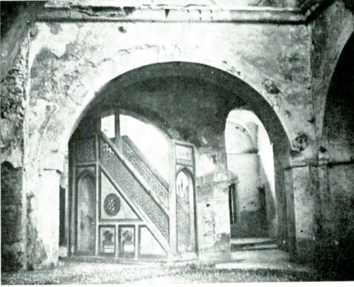
Res. 9 — Merkezi kubbeye mesned teşkil eden kemer ve pilpayeler. Fig. 9 — Piers and arches supporting the central dome.
