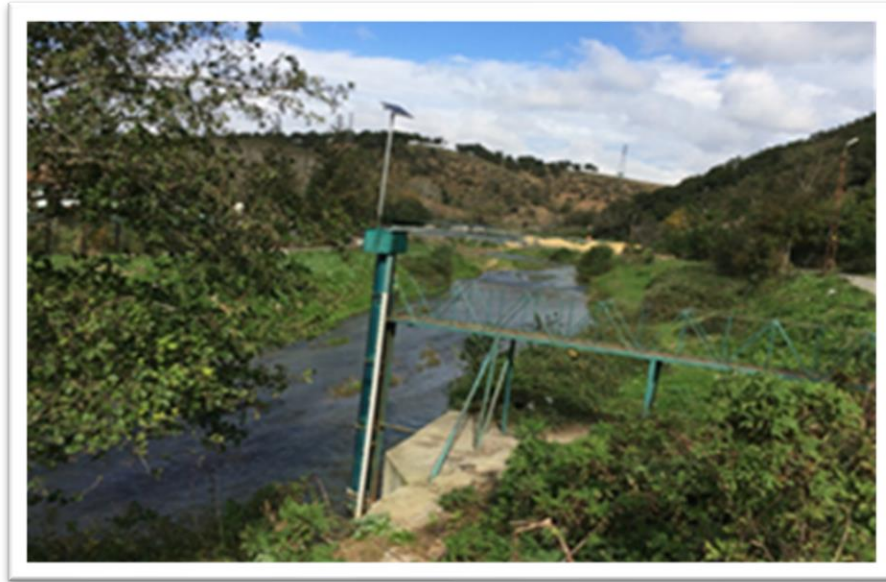
Figure 2. General view of flow meter in Alibeyköy Watershed
