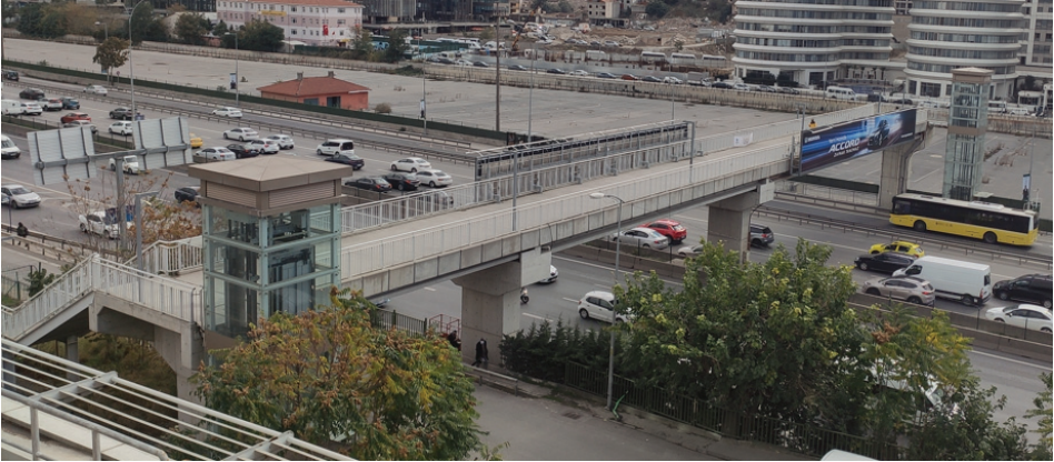
Figure 1 - Studied bridge: Istanbul Medeniyet University pedestrian overpass bridge
