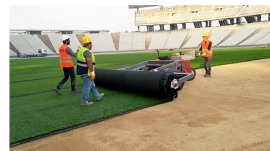
Figure 5. The process of laying the carpet-based 'hybrid carpet'
