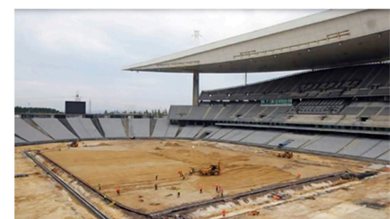
Figure 4. Establishment of the new root zone (Hatko Sport, 2019)
