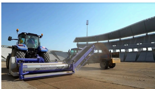
Figure 3. Removing The Existing Natural Grass Surface (Hatko Sport, 2019)
