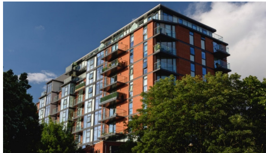
Şekil 5. Battersea Place, Londra (Earth Regeneration, 2023).
