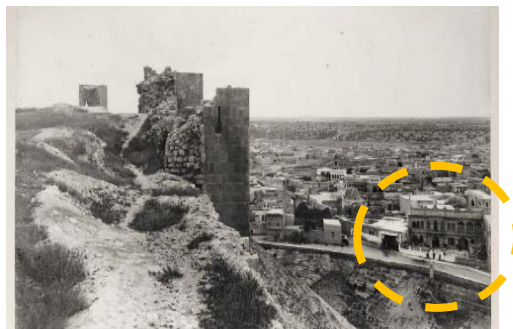
Figure 11. Dar Al-fatwa building.
