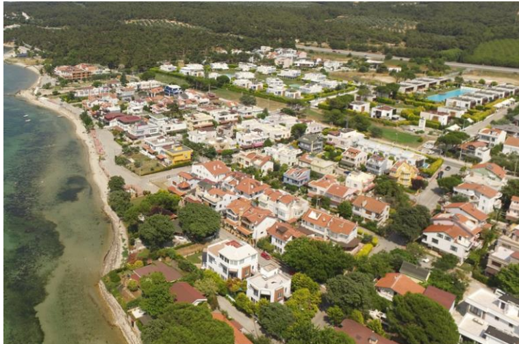
Figure 5. General Facade Views (Original. 2023)
