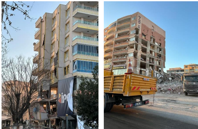
Figure 7. Damaged masonry walls in Adiyaman city center
