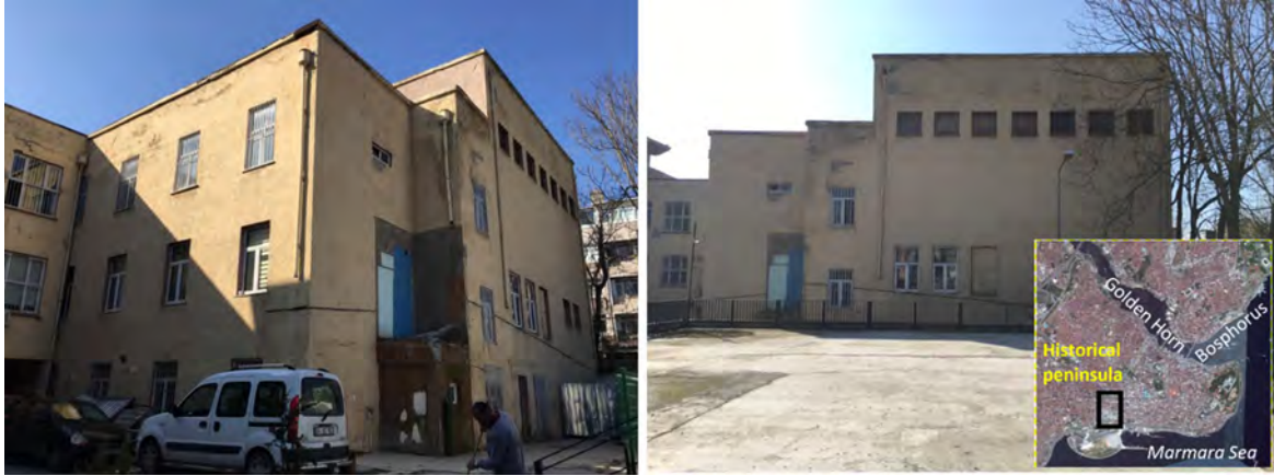
Figure 1. The current condition of the examined building
