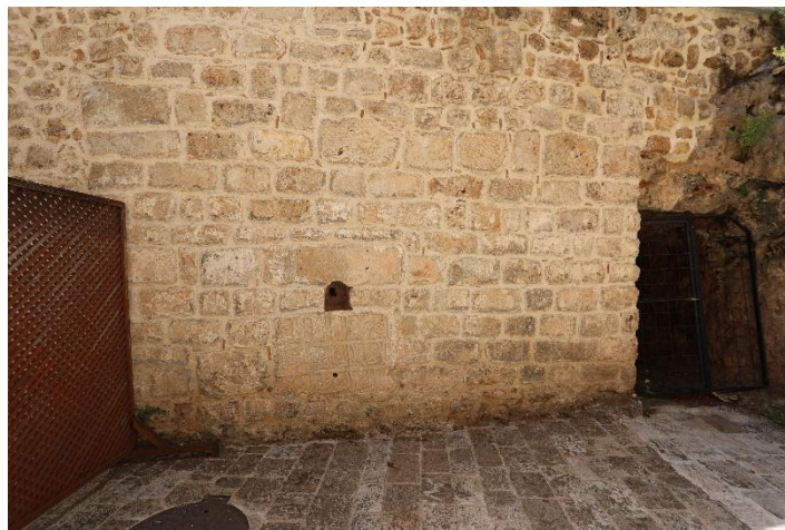
Figure 4. East facade of Yivli Minaret (Mevlevihane) Bath
