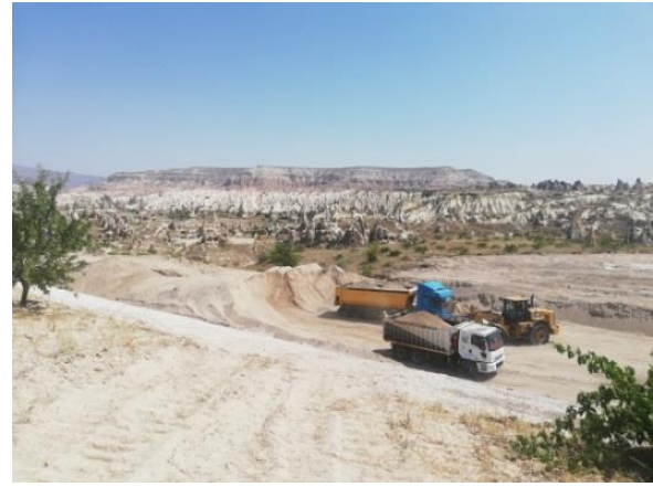
Figure 31. The Saklı Church new vehicle road (Ertürk, 2022)
