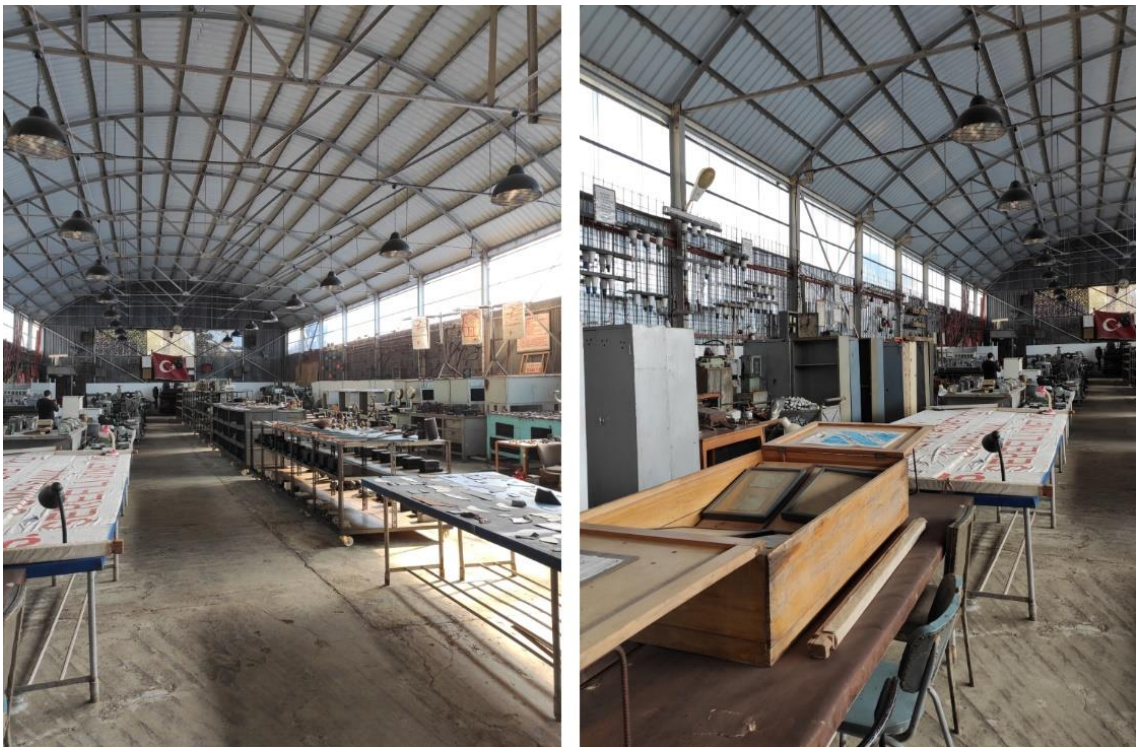
Figure 4. Conservation of the warehouse by providing a function similar to the old function
