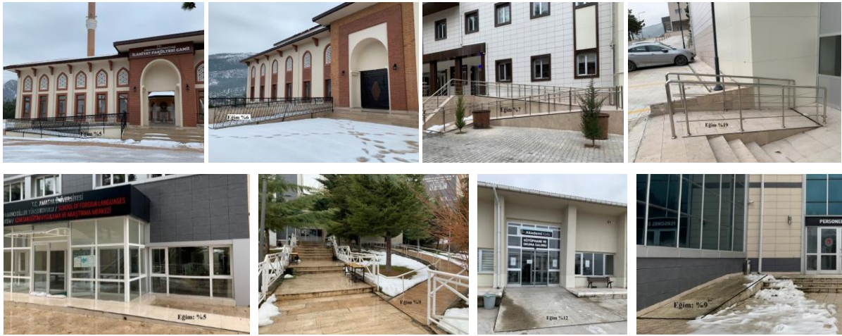
Figure 5. Some ramps near buildings in Yeşilirmak Campus
