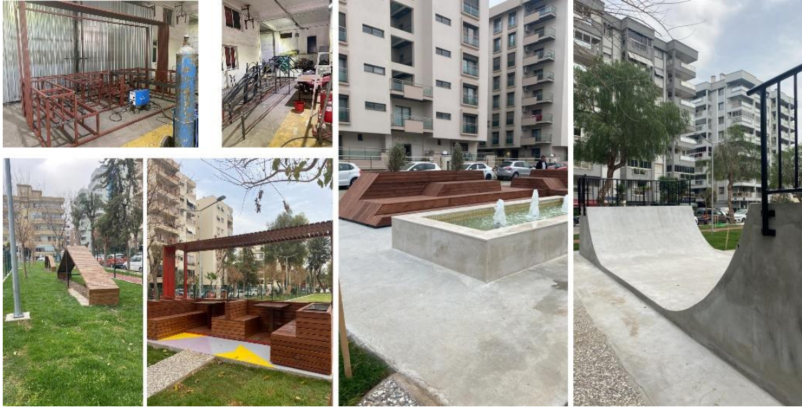
Figure 11. Visuals from the production and on-site implementation of urban elements (Photos: Pelin Özden)
