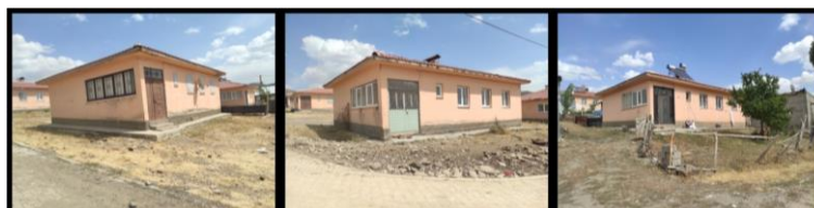
Figure 12. Examples of AFAD houses with enclosed terraces
