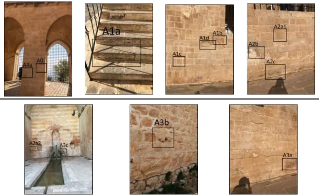
Figure 10. Demonstration of the stones selected for the use of XRF chemical method for the deterioration of Hatuniye Madrasah on the facade
