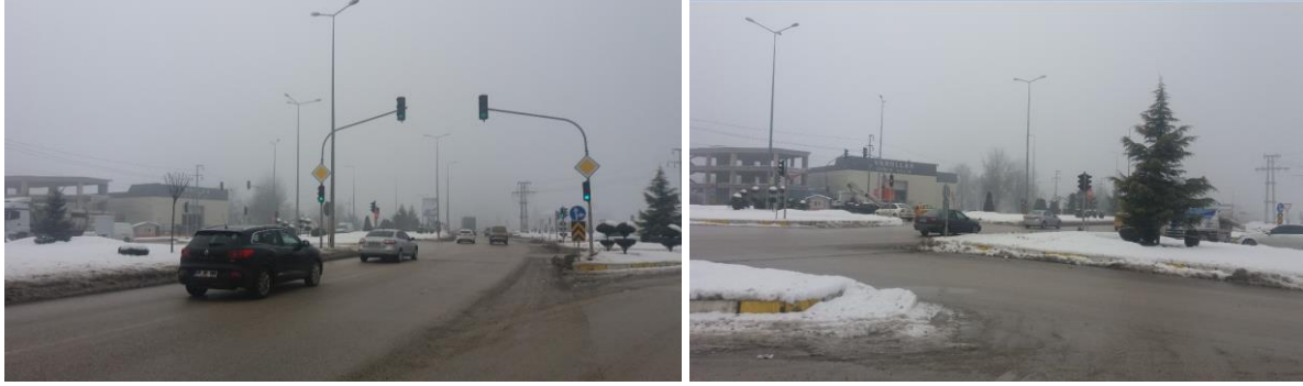
Figure 7. a) View of the intersection, b) the tree that does not allow safe passage and obstructs the view.
