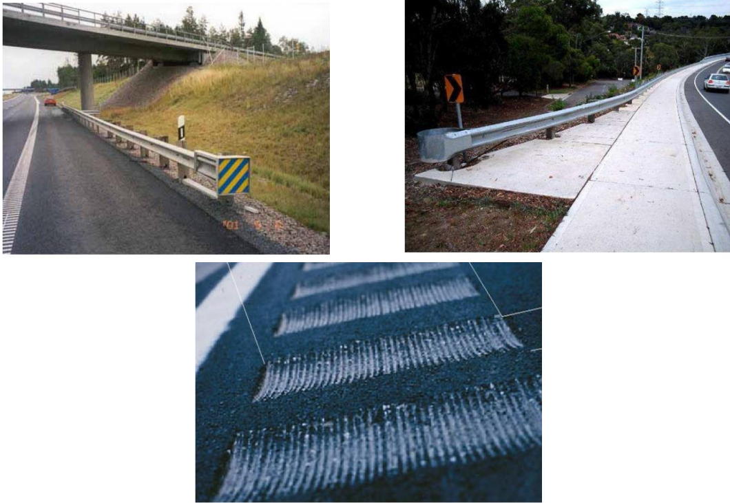
Figure 2. a) Tangent terminal (Thomson et al., 2006b), b) flared terminal of guardrail (La Torre, 2012), c) typical shoulder rumble strip (Thomson et al., 2006b).
