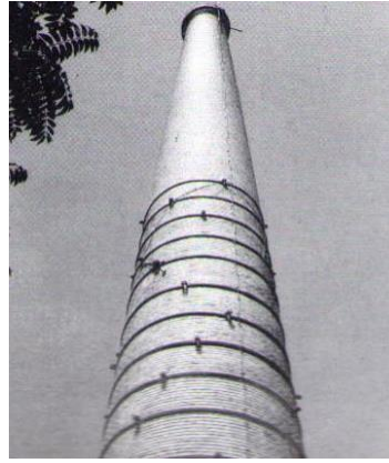
Figure 14. Cooling tower of the complex ( Kheirabadi, 2019 )
