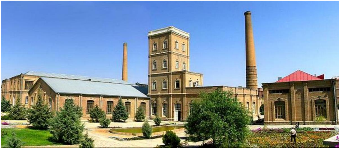
Figure 15. General view of the complex after conservation ( Kheirabadi, 2019 )
