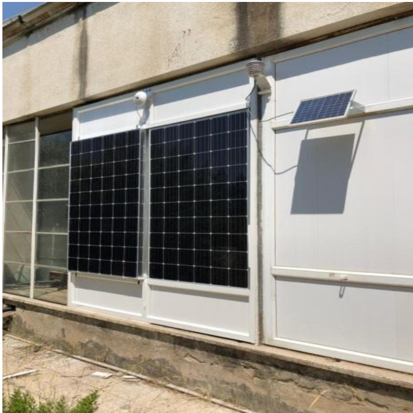
Figure 8. Mounted view of PV/T air collector.
