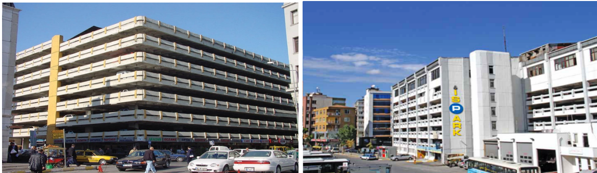
Fig. 6. Existing car parks as potential charging stations [29]
