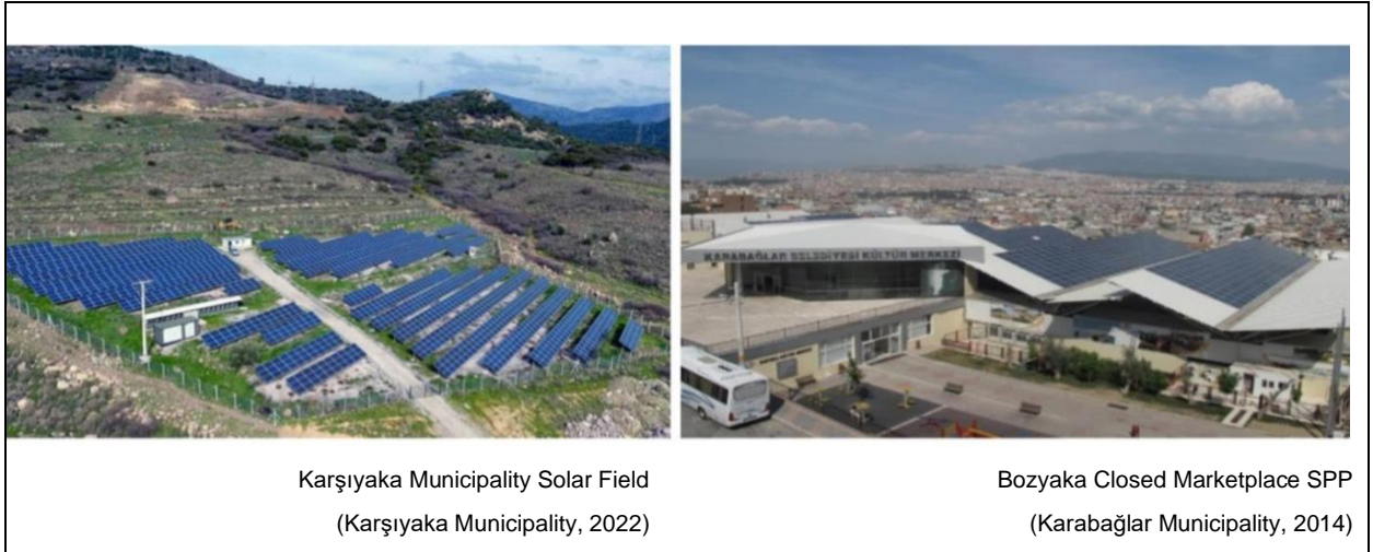
Figure 3. In Izmir, the solar panel belonging to different local municipalities.
