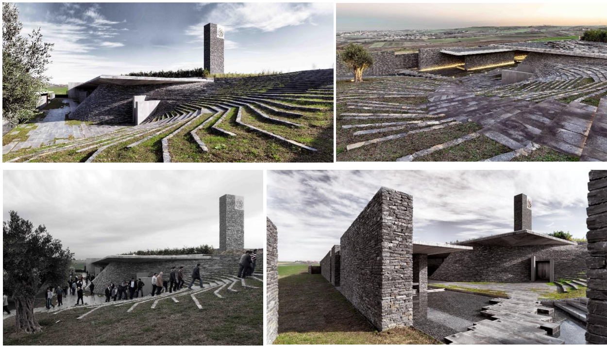
Figure 4. Sancaklar Mosque (Emre Arolat Architects, n.d.)
