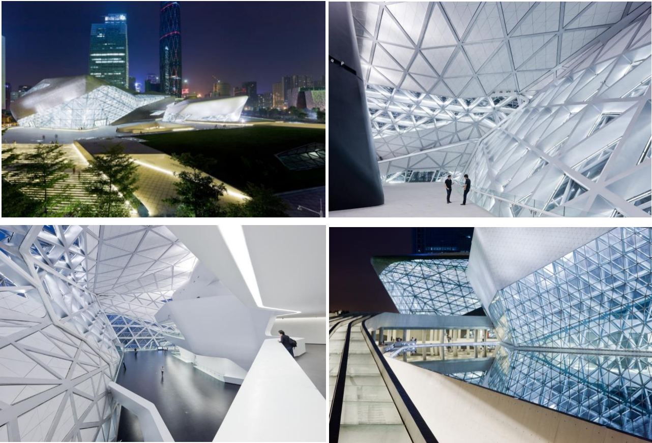
Figure 6. Guangzhou Opera House (Arkitektuel, n.d.)
