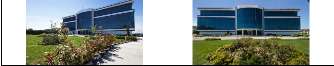
Figure 1. Exterior View of the Existing Pharmaceutical and Vaccine Production Facility
