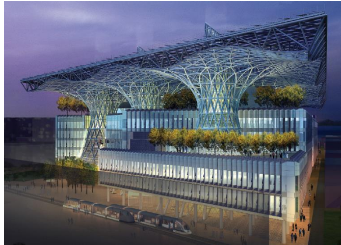
Figure 7. Masdar Headquarters and its roof canopy. Source: Menichetti and van Vuren, 2011
