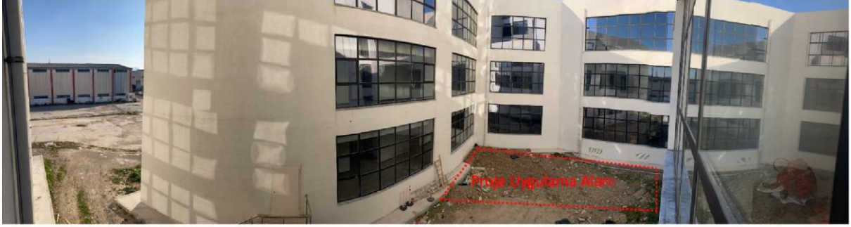
Figure 2. The study site for a rain garden application.
