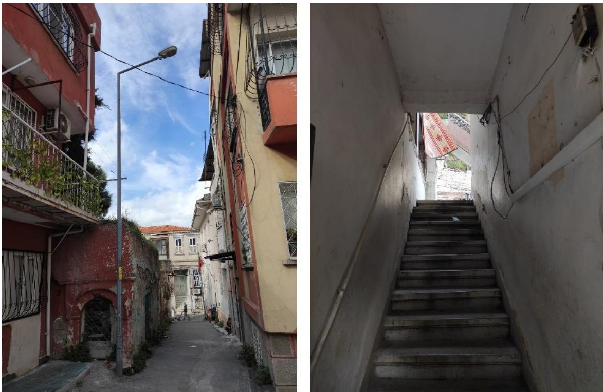
Figure 3. a) (left, corresponds to View 1 on Figure 5). Street view with İplikçi İsmail Dede Tomb cemetery entrance. b) (right, corresponds to View 2 on Figure 6). Courtyard entrance. (Author 1's archive, 2023).
