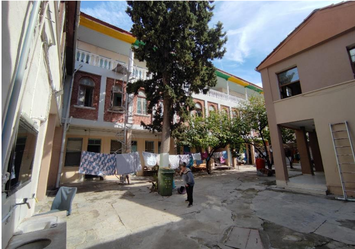
Figure 10. Manisa Akhisar Hotel courtyard general view (Author 1's archive, 2023).
