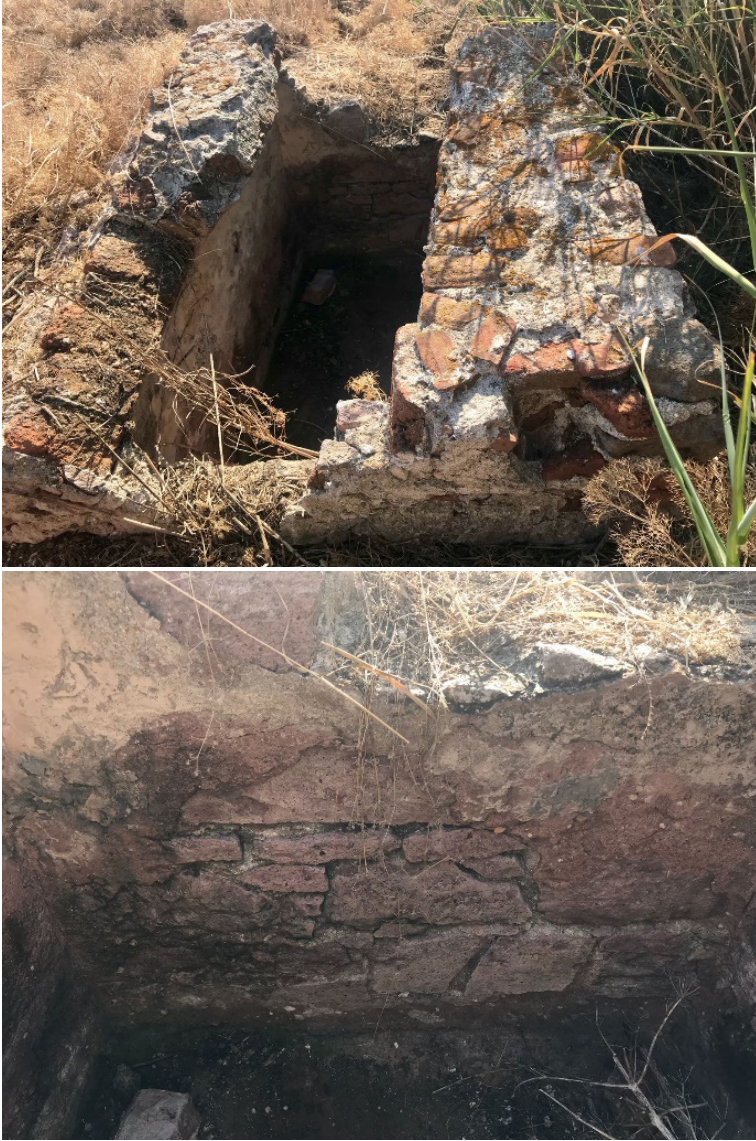
Figures 23–24. Damaged cistern towards the west on Kumru Island (Adramytteion Researches, 2018).
