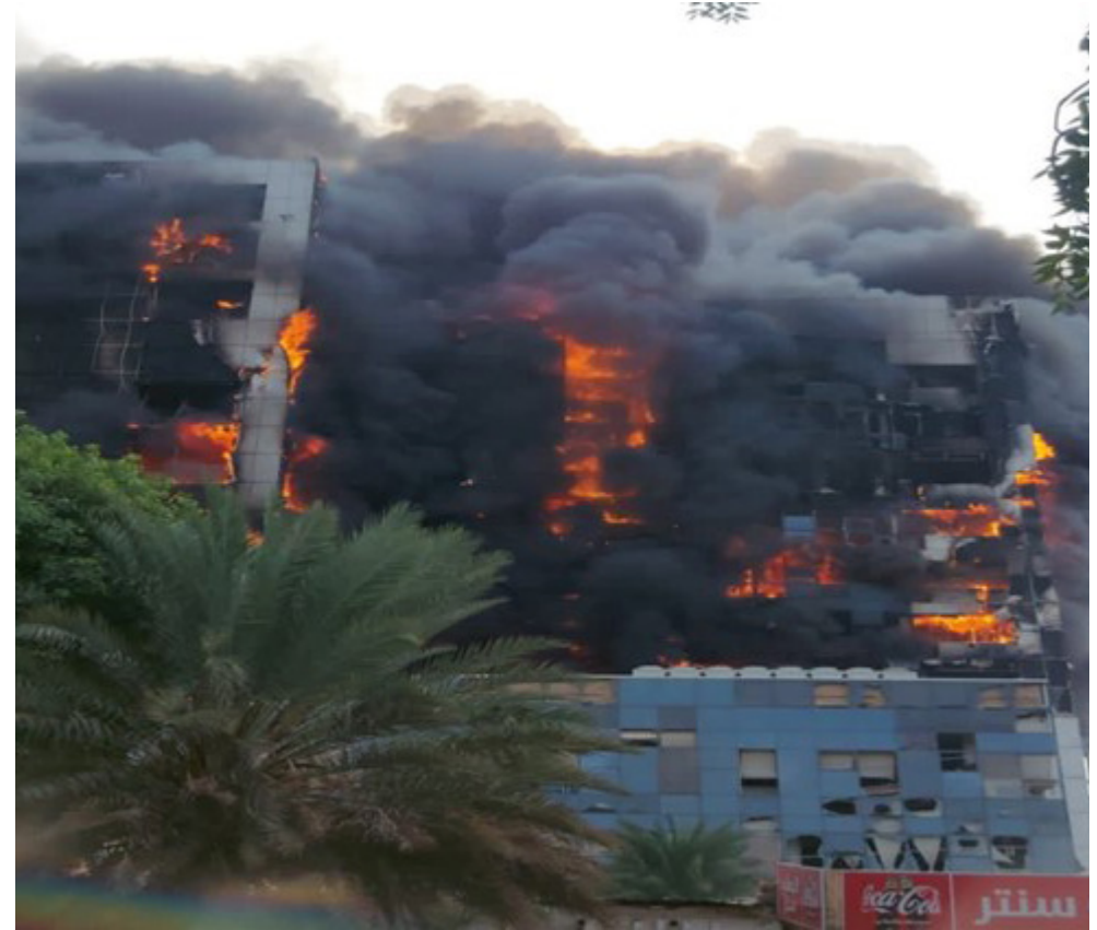
When vitally important sovereign headquarters, including Khartoum International Airport, which is the country's largest airport providing air transportation from the capital Khartoum, became completely unusable because of the attacks of the Rapid Support Forces in the first days of the war, domestic and international flights from here were completely stopped. Due to the military or civilian importance of airports in the war, Khartoum Airport was completely destroyed. The building and airfield were made unusable. Most of the aircraft were destroyed and were completely out of service.
