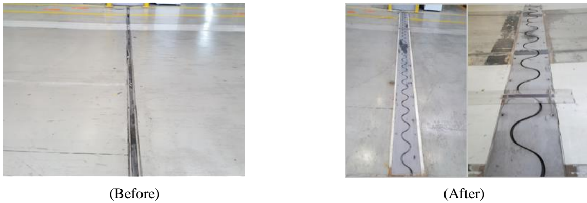
Figure 6. Renewal of concrete slabs
