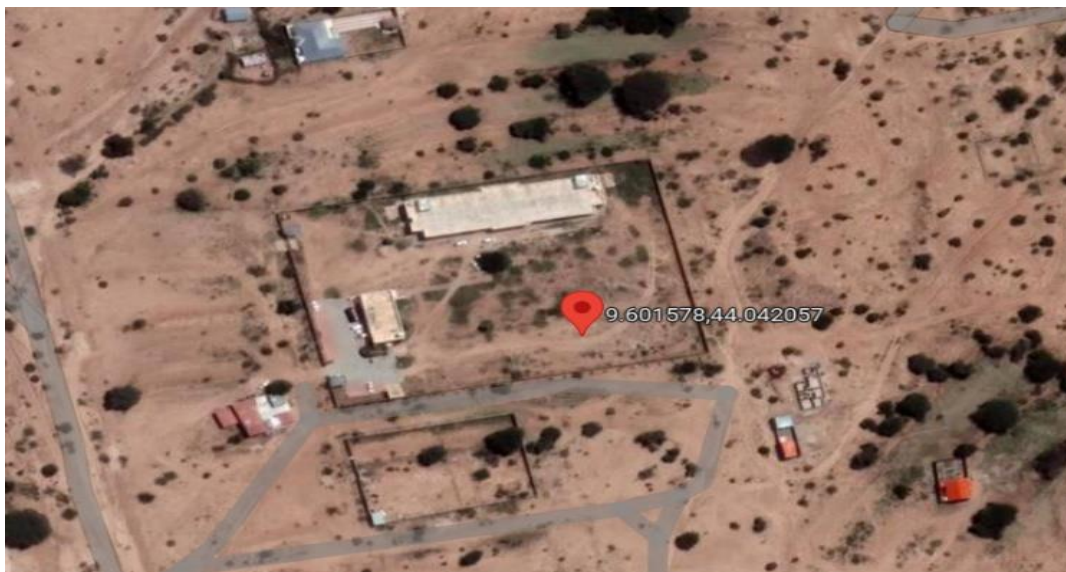
Figure 1. Location of the project on Google Maps showing previously existing buildings
