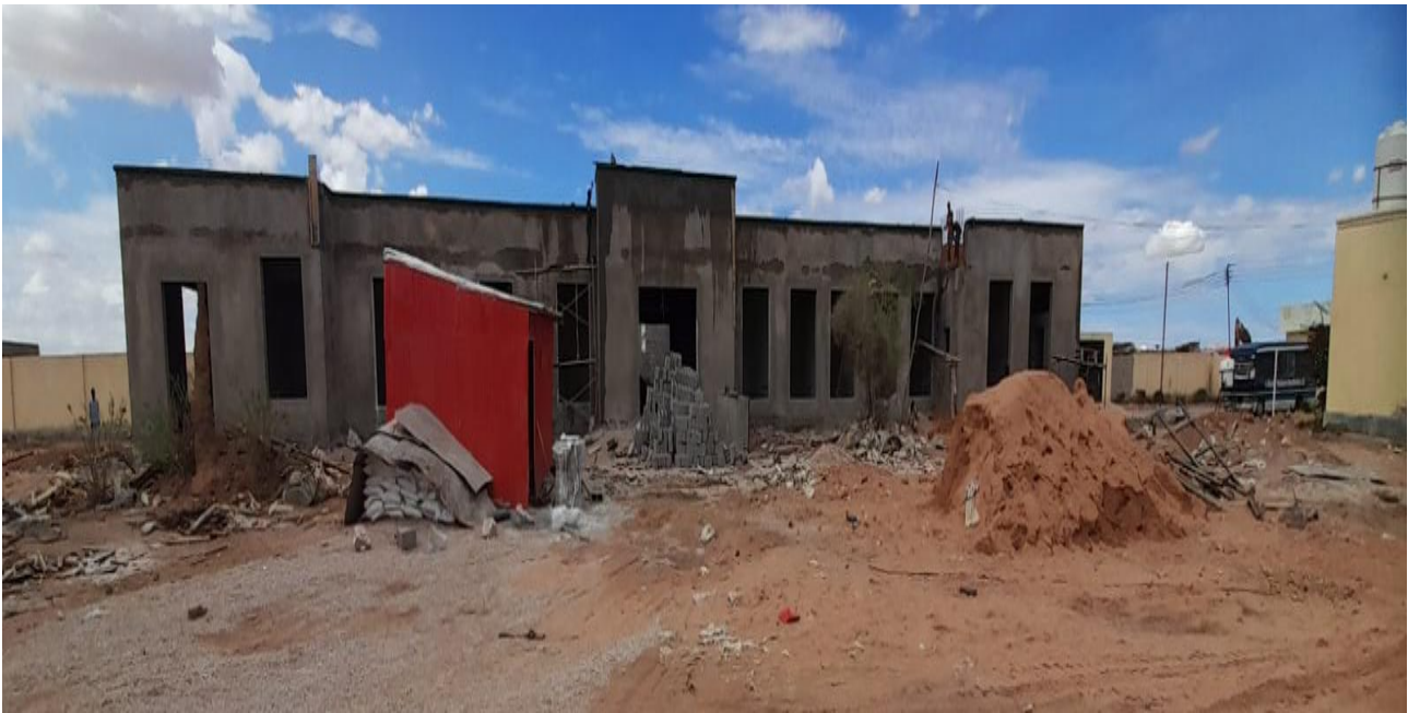
Figure 4. The current stage of the construction
