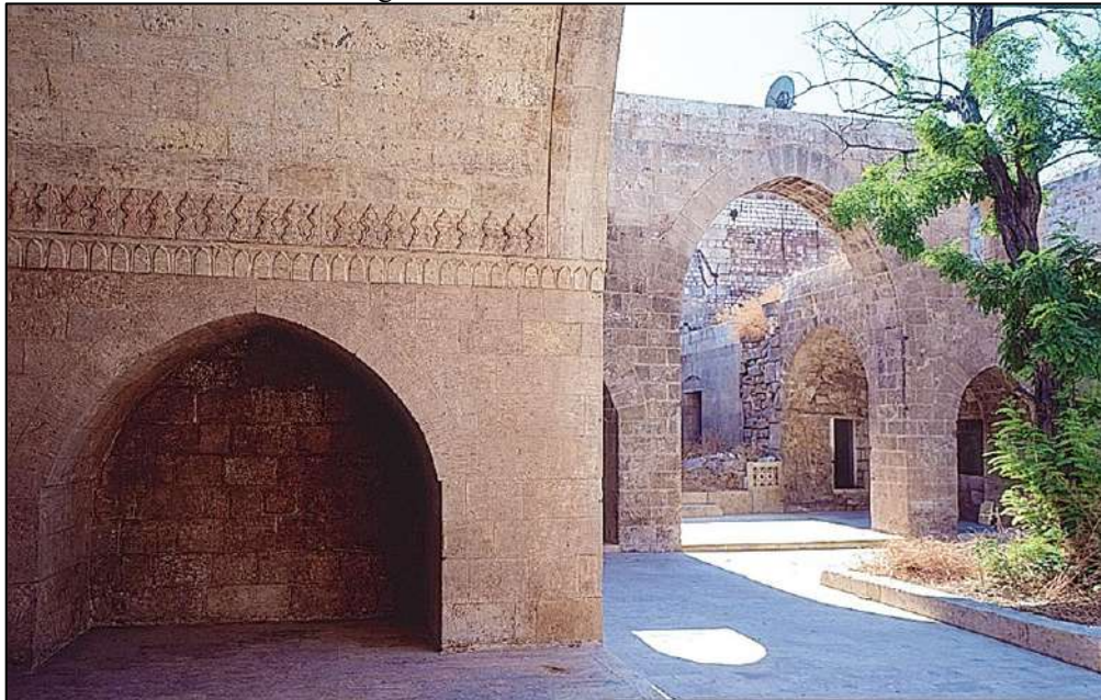
Figure 4. View After Restoration
