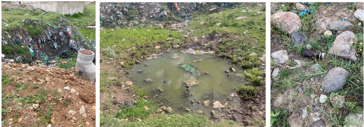
Figure 2. Residue Images from Bingöl Province Old Landfill (May 2022).
