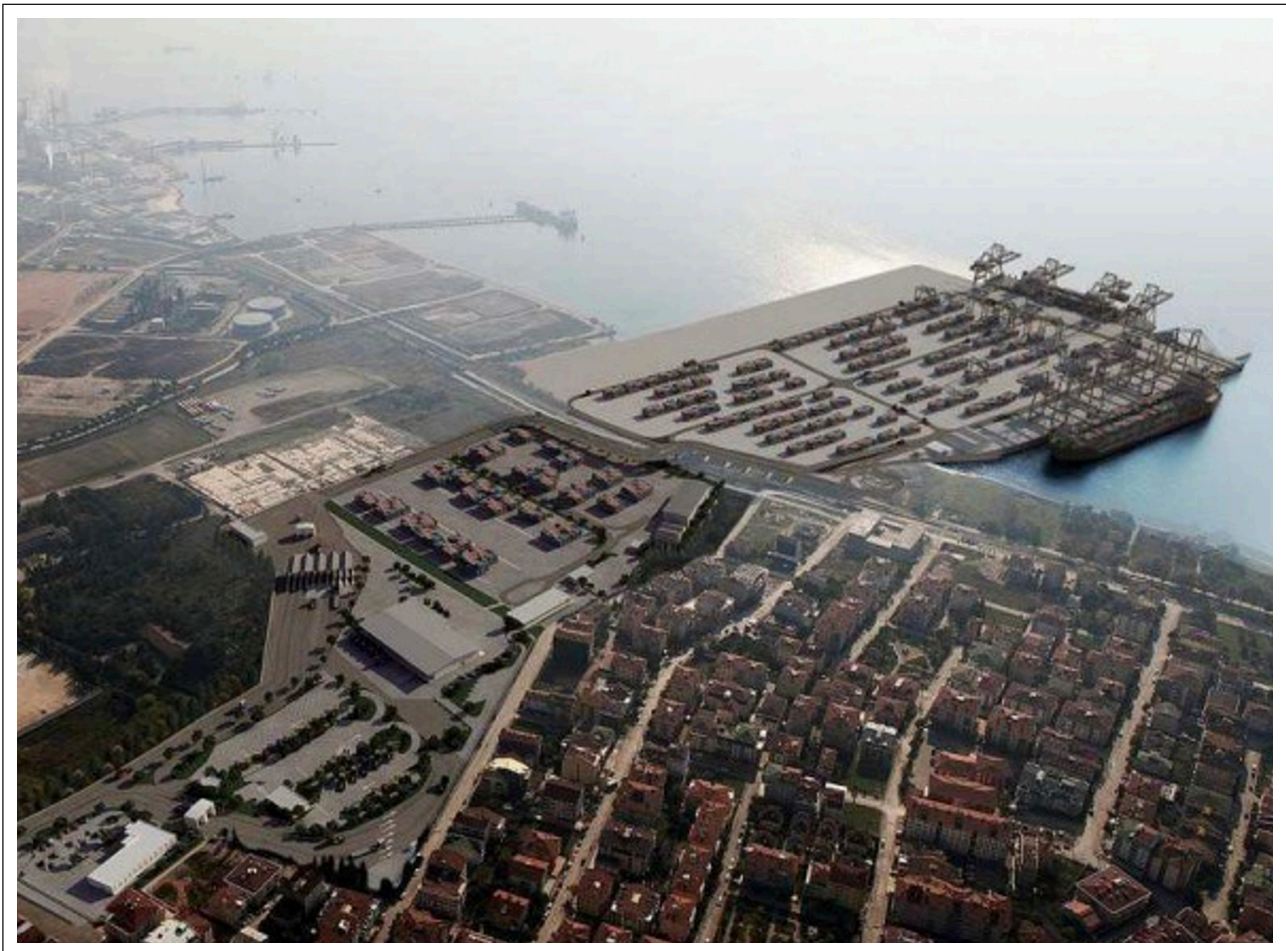
Figure 5. Completed Yarımca container terminal project.
